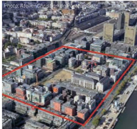
...and during construction.
