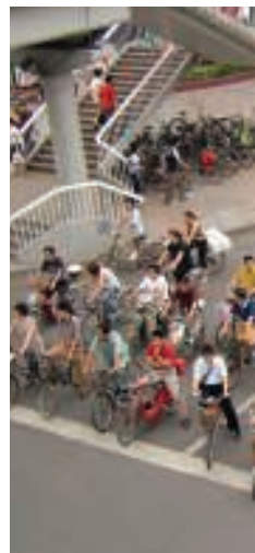
Bollards connected by a white railing protect cyclists from turning right. Cyclists get their own left turn lane in the
