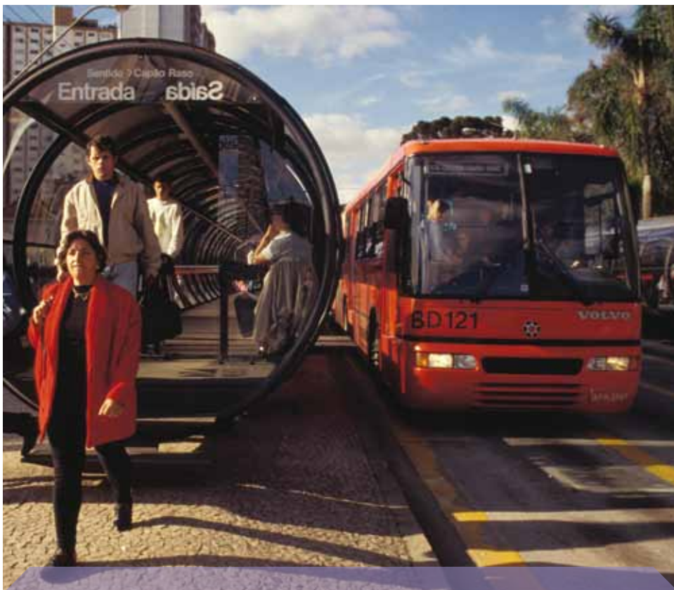
Curitiba, Brazil: a tubular bus station and sleek, modern bus, part of the city's integrated transport system.
